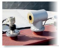
The high temperature type NIVOCAP CMV-115 capacitance level switches are mounted so that the probes sense when the tanks are filled up to 80% and the high temperature type PiloTREK WJS-182 radars are continuously measuring the level of the hot bitumen. Upon reaching the high level during filling of the tank the NIVOCAP CK level switches send switching signals to the sound and visual alarm devices to warn the personnel to stop the filling.
